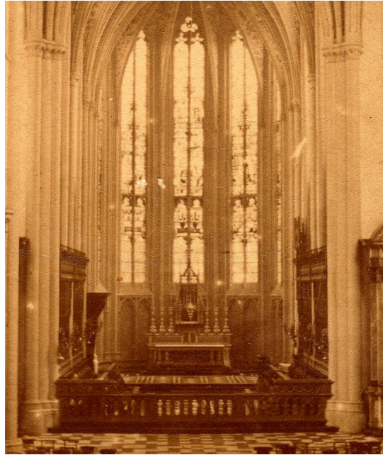
Figure 6 A view circa 1870 of the main altar showing the temporary altar which was retained until 1881.
